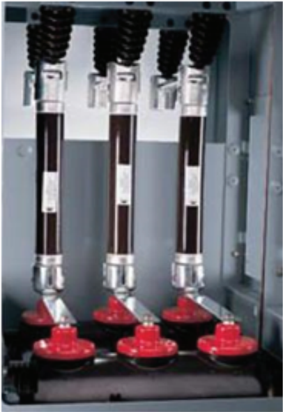
Figure 66 - Current-limiting Power Fuses and Mountings
