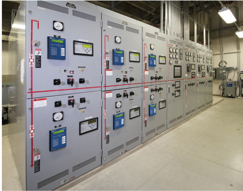
Figure 125 - Three-Generator Medium Voltage Emergency/Standby System
