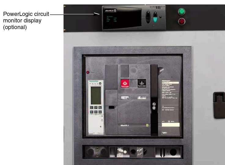
Figure 39 - PowerLogic Circuit Monitor Display
