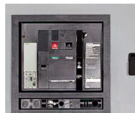
Figure 6 - Through-the-Door Access
