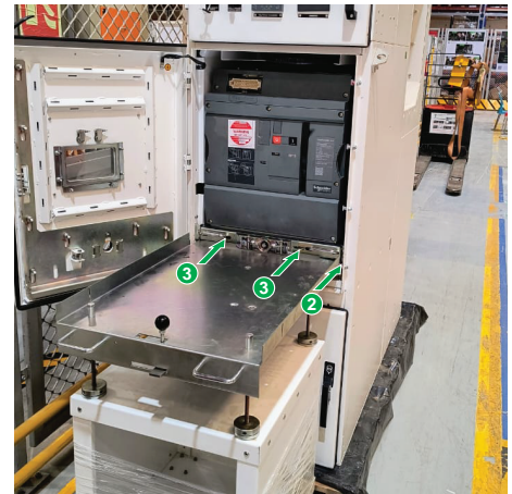
Figure 24 Locking Transport Trolley on Panel
