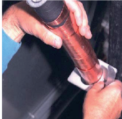
Figure 44 Cut rubber sleeves to size and slip them onto the cables
