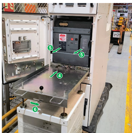
Figure 25 Coupling the Transport Trolley to Panel
