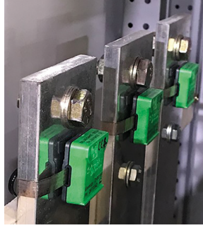
Connection Temperature Monitoring
