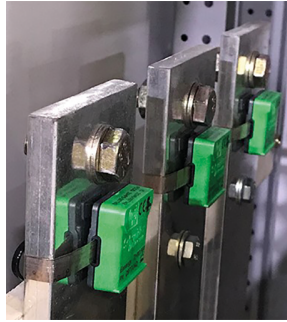
Connection Temperature Monitoring
