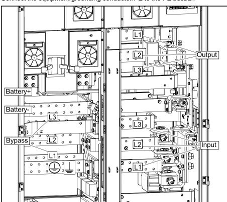
2. Connect the equipment grounding conductor/PE to the PE busbar.
