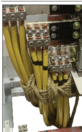
Figure 55 - Cable Restraint Examples
