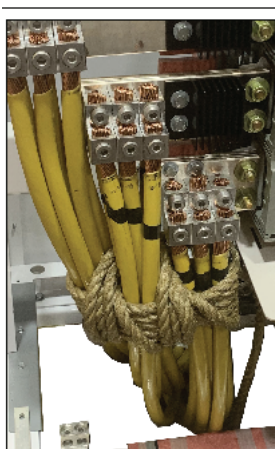
Figure 62 - Cable Restraint Examples
