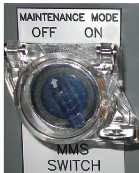
Figure 60 - Commutateur MMS
