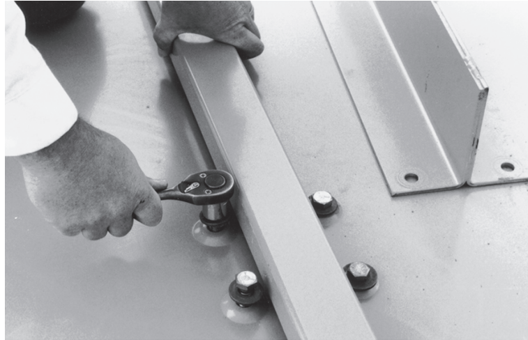
Figure 11 - Plugging Holes with Bolt/Seal Washers
