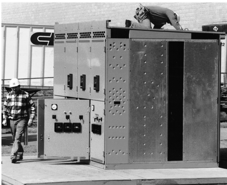
Figure 7 - Securing Switchgear Sections
