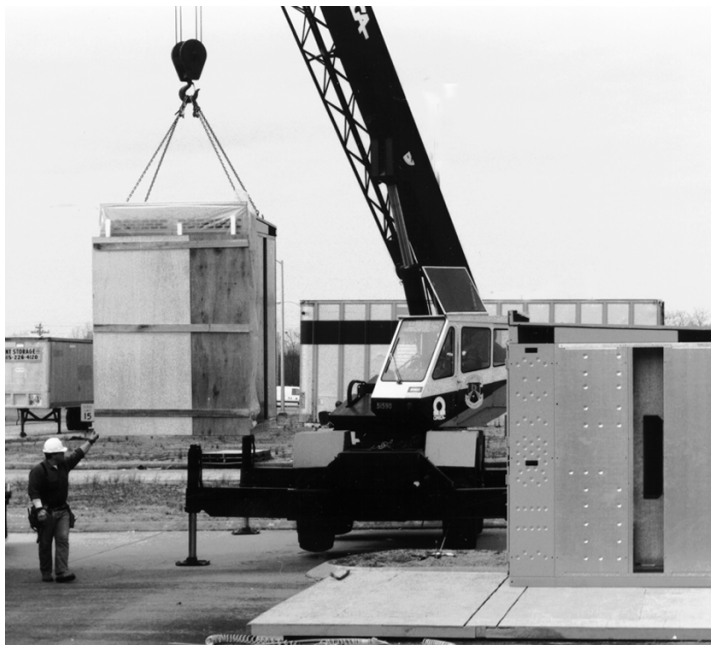
Figure 6 - Unloading Second Section
