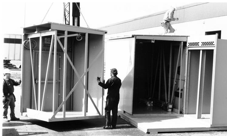
6. Using a crane, set the second aisle section onto the concrete pad approximately 12 inches (305 mm) from the section in place.
