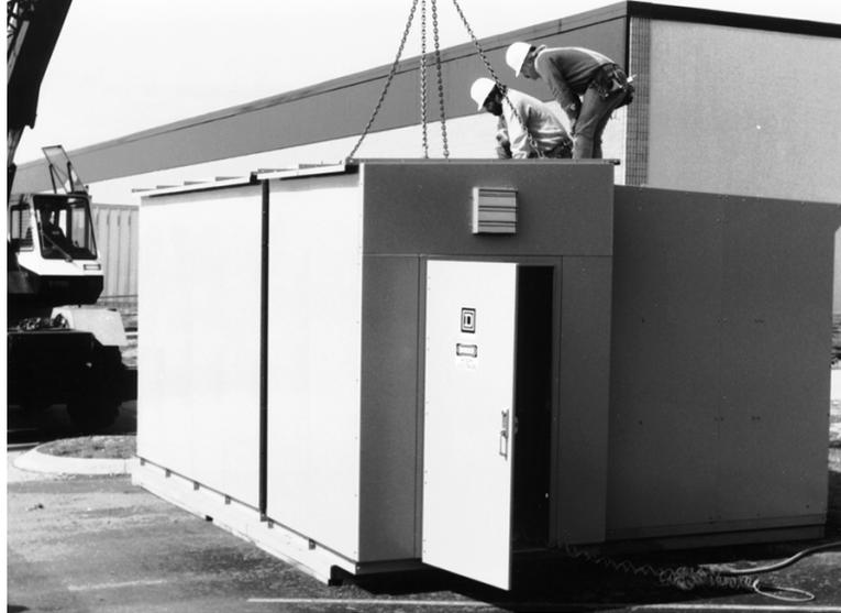
8. Install, level, and attach the second aisle section to the switchgear by bolting each bay's aisle roof support bracket to the front of switchgear, and by bolting the aisle roof to the switchgear roof. Use steel shims, if necessary, to make sure there is an alignment.
