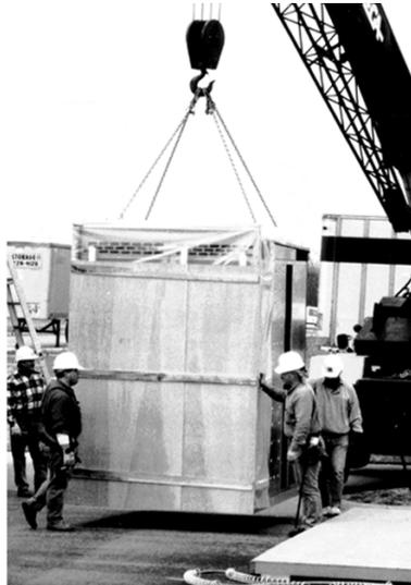
3. Remove the shipping covers. Be careful not to damage the instrumentation on the front doors when removing shipping covers.
