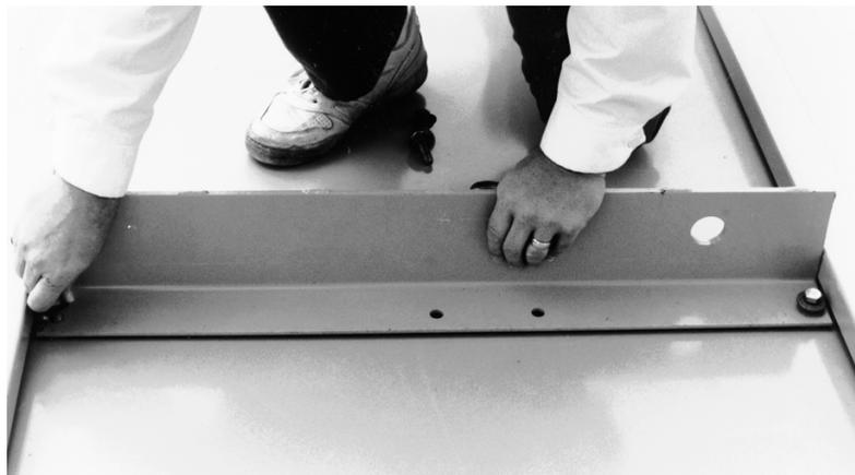
**Figure 23 - Removing Small Lifting Lugs**
