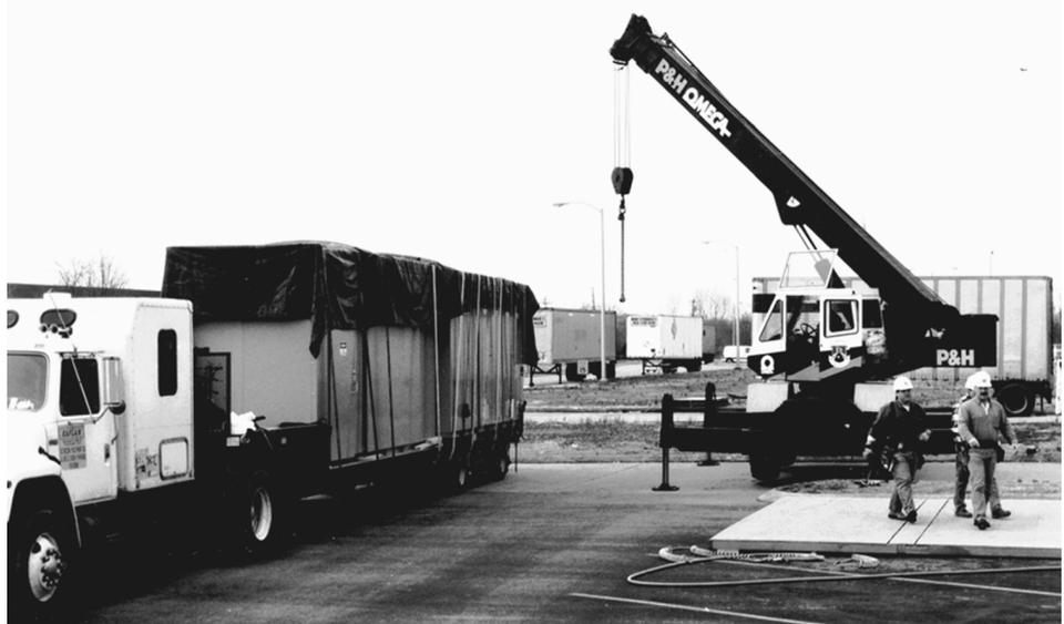
2. Unload the switchgear shipping sections from the delivery truck. The shipping sections are designed to be lifted by a crane. Attach a sling to the lifting lugs on the roof of each of the shipping sections as shown in . A spreader bar may be necessary to maintain proper lifting angles. If a crane is not available, contact Schneider Electric for special arrangements for unloading the switchgear sections.
