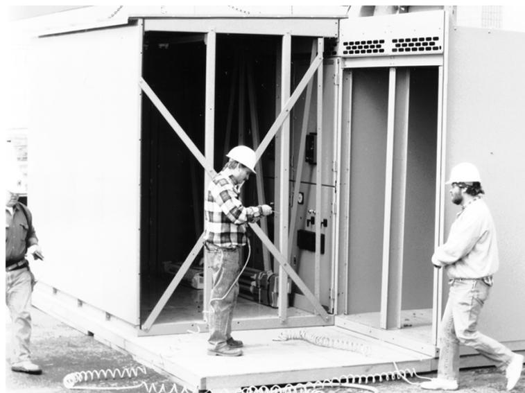
3. Attach the aisle section to the switchgear by bolting each bay's aisle roof support bracket to the front of the switchgear and by bolting the aisle roof to the switchgear roof, using the supplied 3/8-16 x 1.0 inch bolts (Anchoring Aisle Roof Support Bracket to Switchgear, page 24).
