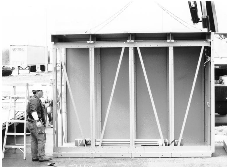
2. Verify that the vertical sections, the base, and the roof are aligned with the switchgear shipping sections. Use steel shims if necessary. It is important that the bolt holes on the aisle roof support brackets align with the corresponding holes on the front of switchgear sections.
