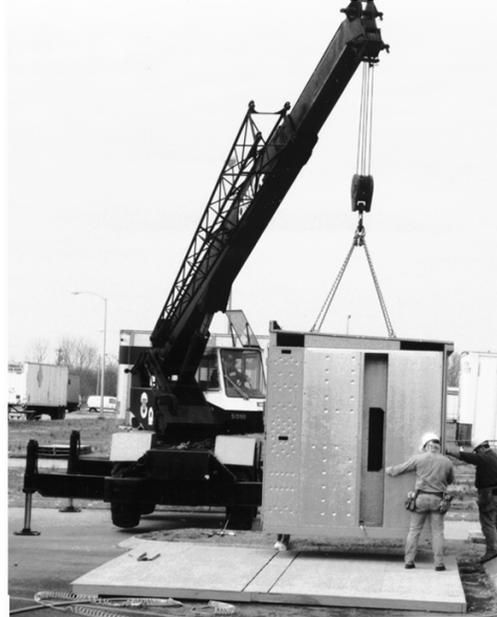
5. Level the switchgear shipping section using steel shims if necessary.
