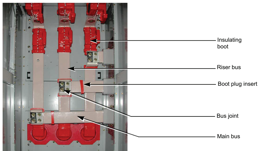
Figure 26 - Main Bus (with rear bus cover removed)
