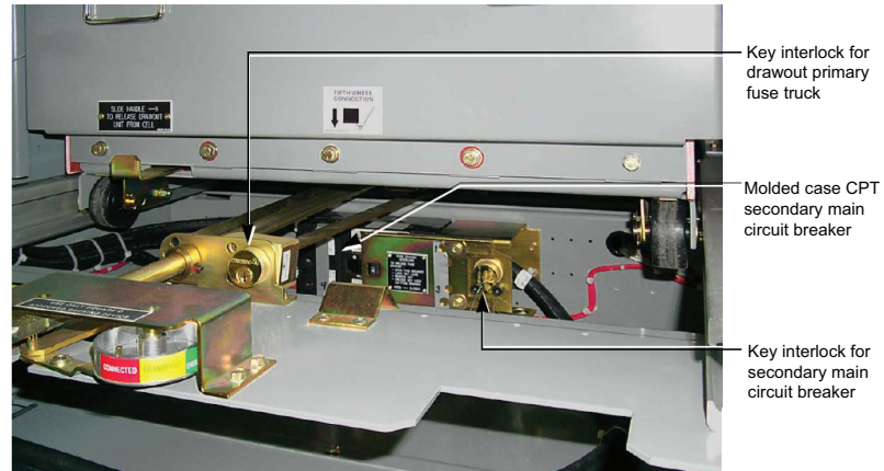
Figure 28 - Key Interlocks for Drawout Primary Fuses and Secondary Circuit Breaker
