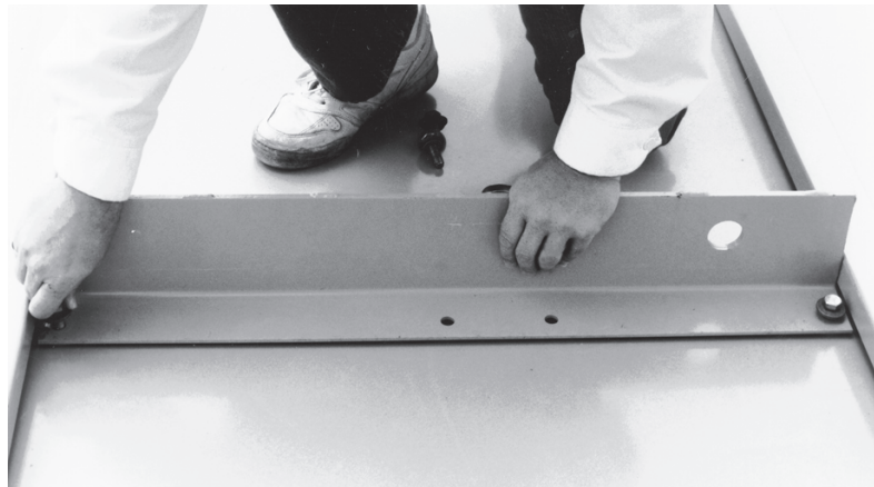
Figure 9 - Removing Small Lifting Lugs
