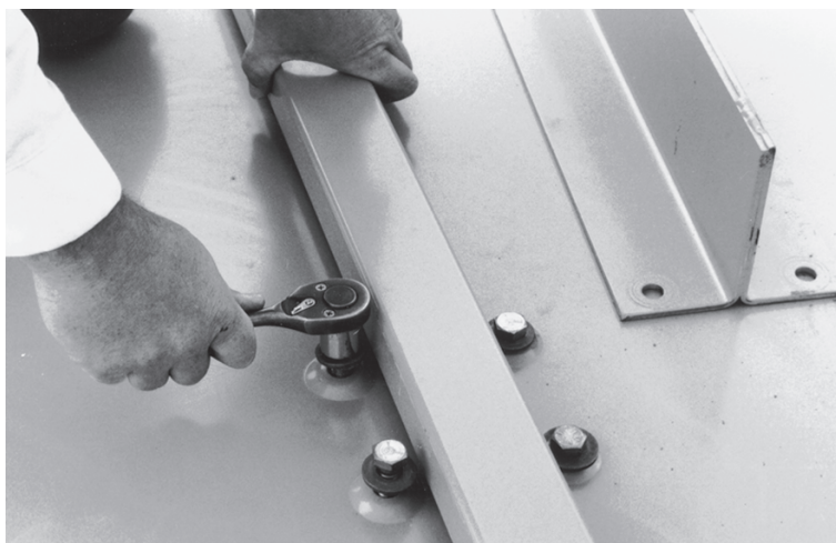
Figure 10 - Plugging Holes with Bolt/Seal Washers
