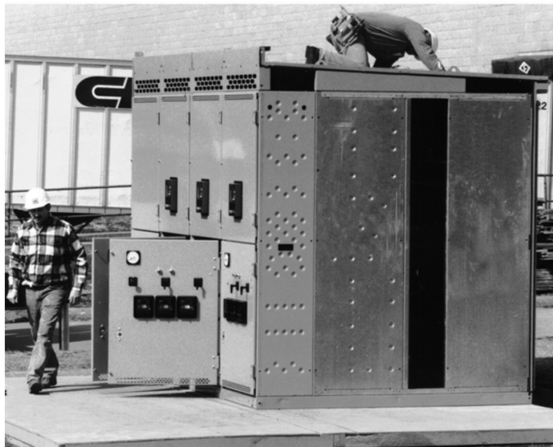
Figure 6 - Securing Switchgear Sections
