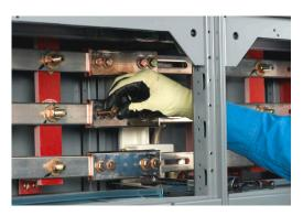
Figure 45 - Place a Conical Washer Under the Bolt Head
