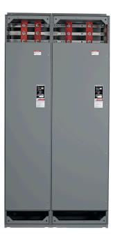
View C: Two-piece Bus Barriers Removed (splice connection made)
