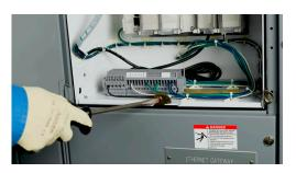
5. Disconnect the power wiring from the starter terminals or, if provided, the power terminal blocks. Tag the terminations for re-installation (see Disconnected Terminal Blocks, page 124).
