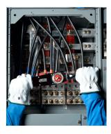
Connection Torque Values for Main Lug Compartments and Connection Torque Values for Main and Branch Feeders provide main disconnect and branch feeder torque values, which apply to both aluminum and copper conductors.
