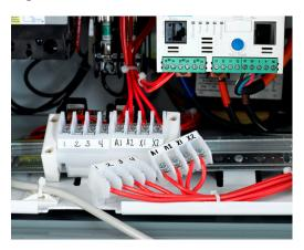
6. Push the power leads and the top portion of the control pull-apart terminal blocks through the wiring port and into the vertical wireway (see Power Leads and Top of Terminal Blocks Fed Through Wiring Port, page 124).
