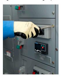
4. Check for live circuits using a properly rated voltage sensing device. De-energize any voltage sources.
