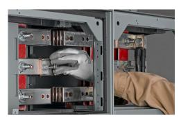
Figure 58 - Place a Conical Washer Under the Bolt Head
