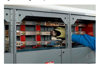
3. Reinstall the two left bolts through the splice bars and into the horizontal bus (see Insert the Splice Bolts, page 63); make sure the original conical washers are reinstalled with the concave side facing the splice bus (see Place a Conical Washer Under the Bolt Head, page 63).
