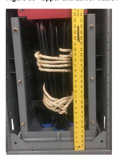
7. Make sure the cable bundles do not disengage the interphase barriers from the grooves of the ArcBlok lug cover (see ArcBlok Interphase Barriers, page 94 and ArcBlok Interphase Barriers and Lug Cover Grooves, page 95).
