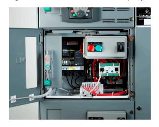
Figure 157 - TeSys T Controllers
