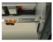
3. Slide the ground splice bar into the right section, aligning the mounting holes (see Ground Bar Bolt Replaced, page 72).
