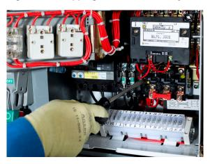
**Wiring and Electrical Connections**: Verify that all electrical connections are correct; tighten them if necessary (see Tightening Electrical Connections, page 133). For any inaccessible electrical connections, contact Schneider Electric Services. Also inspect
