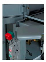
If the withdrawn unit is left in the structure, use appropriate lock-out procedures to avoid re-loading by non-authorized personnel (see Locked Out Device, page 125).
