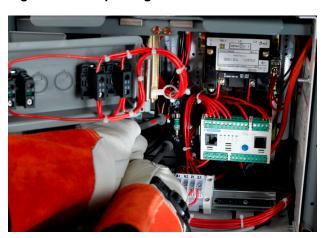
**Starter Contacts**: Check the starter contacts (see Starter Contacts, page 132). Replace any that are badly worn or pitted. (See the Schneider Electric Literature Lists, page 12 for the appropriate instruction bulletin.)
