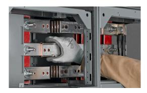
Re-install the two left bolts through the splice assembly and into the horizontal bus (see Insert the Splice Bolts, page 66). Make sure the original conical washers are reinstalled with the concave side facing the splice bus (see Place a Conical Washer Under the Bolt Head, page 66).
