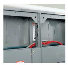
Control and power wires are routed to each unit via the vertical wireway. When supplied, grommeted wire ports must be opened to route wire to the unit. The H-shaped cut pattern is pre-scored for easy opening. Using a small knife, cut through the center tabs and complete the H-shaped slice (see Vertical Wireway Grommet, page 107). When cutting, be sure not to damage the wires located near the grommet.
