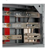
Remove all four bolts from the integral splice bar (see Remove Bolts from Singlesplice Bar, page 60).
