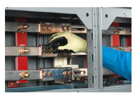
Figure 52 - Place a Conical Washer Under the Bolt Head
