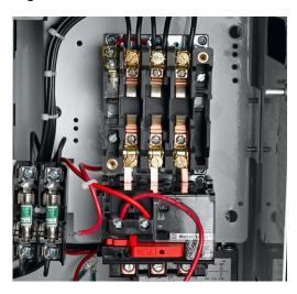
**Control Devices**—Check for proper operation of starters, relays, timers, and other control devices (see Control Devices).
