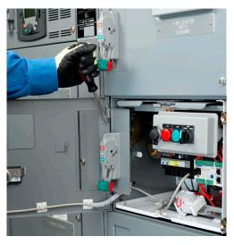
12. When reinstalling a hinge pin, make certain that the hooked end is fully engaged into the hinge collar.
