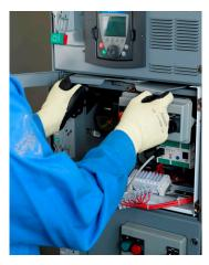
b. Press the handles inward until they are flush with the face of the MCC (see Handles Flush with the Front of the MCC, page 185).
