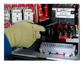
**Starter Interlocks**: Check the mechanical interlocks on reversing, multispeed, or reduced voltage starters.
