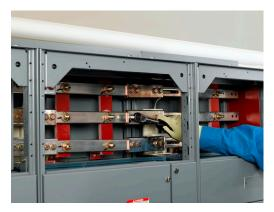
2. Slide the splice assembly to the left until the two left holes are in line with the corresponding holes in the horizontal bus on the left section (see Align the Splice and Bus Holes, page 62).
