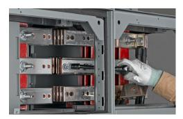
4. Slide the splice assembly to the left until the two left holes are in line with the corresponding holes in the horizontal bus on the left section (see Align the Splice and Bus Holes, page 68).
