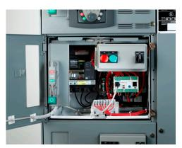
**Overload Relay**: Manually trip the overload relay to help ensure proper operation (see Tripping the Overload Relay, page 132). Verify that the thermal unit is the proper size for the application. Refer to the thermal unit selection tables (Thermal Overload Unit Selection, page 196).
