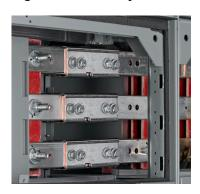
3. Remove all four bolts from each splice assembly (see Remove the Bolts from the Splice Assembly, page 68).
