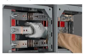
Reinstall all four bolts through the splice assembly and into the horizontal bus (see Insert the Splice Bolts, page 69). Make sure the original conical washers are reinstalled with the concave side facing the splice bus (see Place a Conical Washer Under the Bolt Head, page 69).
