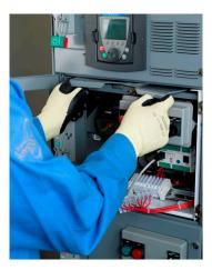
8. The operator mechanism-to-structure interlock helps prevent the control unit from being withdrawn or inserted with the handle in the **ON** position (see Operating the Mechanism-to-Structure Interlock, page 125).
