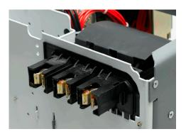
**Circuit Breaker or Disconnect Switch**: Verify proper operation of the circuit breaker or disconnect switch. Inspect switch blades; if evidence of arcing or excessive heat is present, replace the switch assembly. Exercise the push-to-trip feature on the circuit breakers.
