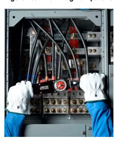
8. Inspect all insulators, braces, and barriers; replace any that show signs of arcing damage, tracking, excessive heat, or cracking.
