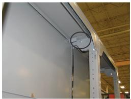
View D: Top Rear Side Channel Connection (Shown with MCC back plates removed.)
