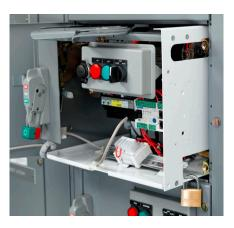
10. Remove the control unit from the structure for servicing (see Control Unit Removed, page 126). In units with a full bottom plate, additional accessibility to the components and wiring can be achieved by folding the bottom plate down. To do so, lean the unit on its back, remove the two front screws, and fold the bottom plate down (see Control Unit with Bottom Plate Folded Down, page 126).
