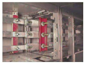
4. Slide the splice assembly to the left until the two left holes are in line with the corresponding holes in the horizontal bus in the left section (see Slide the Splice Assembly to the Left, page 65).
