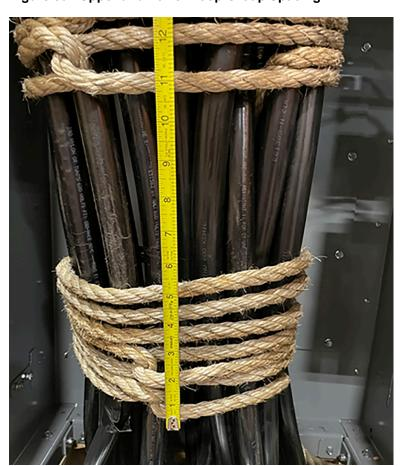
Figure 89 - Upper and Lower Loop Group Spacing
