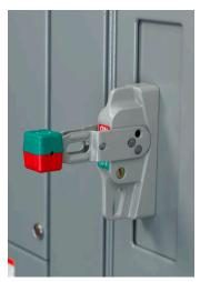
Test for proper **ON**, **TRIP**, **OFF**, and **RESET** positions (F-, K-, and L-frame circuit breakers) or **ON**, **TRIP**, and **OFF** positions (B-, H-, J-, M-, or P-frame circuit breakers). Verify proper door interlock operation.
