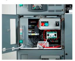
c. Turn the screw on the control unit lock-in panel (when supplied) located at the bottom front of the control unit (see Tightening the Control Unit Lock-in Panel, page 185), until the lock-in pawl is latched to the support shelf below the control unit.
