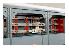
3. Remove the two left bolts from each splice assembly. Then loosen, but do not remove, the two right bolts of each splice assembly (see Loosen Bolts, page 65). If the bus has optional 85,000 A bus bracing supplied (see 85,000 A Bracing Option, page 65), also loosen the center nut of each splice assembly.
