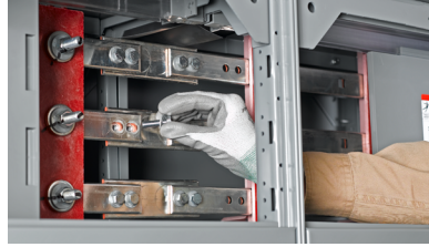
Figure 38 - Place a Conical Washer Under the Bolt Head
