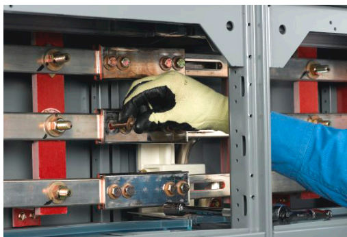
Figure 43 - Place a Conical Washer Under the Bolt Head
