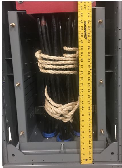
Figure 70 - Upper and Lower Cable Lacing Groups
