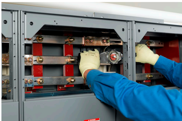
Figure 44 - Torque the Bolts
