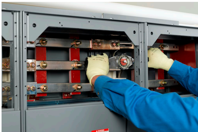
Figure 51 - Torque All Bolts
