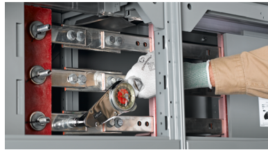
Figure 39 - Torquing the Bolts
