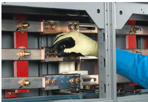
Figure 50 - Place a Conical Washer Under the Bolt Head
