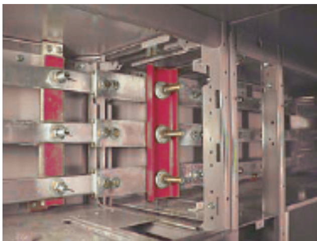
Figure 47 - 85,000 A Bracing Option
