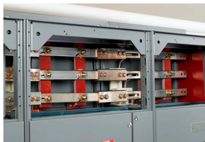
Figure 45 - Wireway Covers Removed and Horizontal Bus Barriers Open
