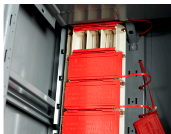
Figure 144 - Removing the Manual Bus Shutter
