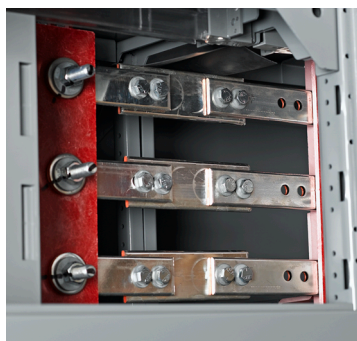
Figure 33 - Correct Application of Splice (shown installed) for 600/800 A, Non-Fork Bus
