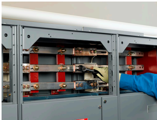
Figure 40 - Remove the Left Bolts and Loosen the Right Bolts on the Splice Assembly
