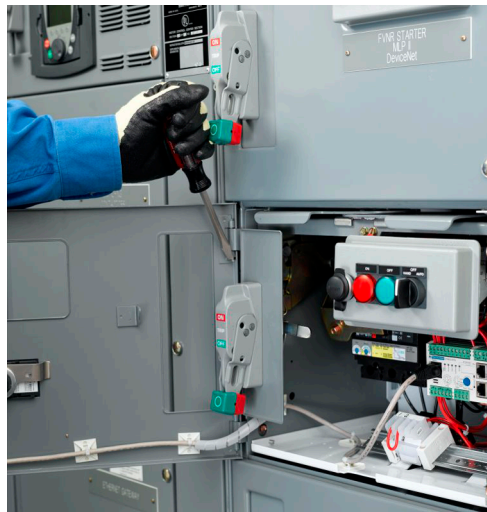
Figure 105 - Driving Out Hinge Pin
