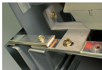
Figure 61 - Ground Bar Bolt Replaced
