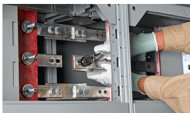
Figure 35 - Remove Bolts from Single-Splice Bar
