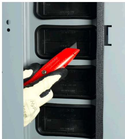
Figure 143 - Cutting the Vertical Wireway Grommet (when supplied)
