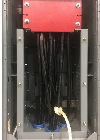
Figure 69 - First Cable Lacing Loop
