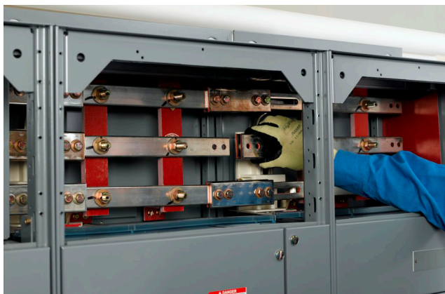
Figure 41 - Align the Splice and Bus Holes
