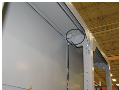
View G: Top Rear Side Channel Connection (Shown with MCC back plates removed.)
