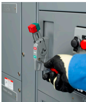
Figure 120 - Operating Door Interlock Defeat Mechanism
