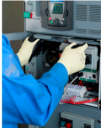
Figure 100 - Pulling the Twin Handle Cam Mechanism Forward
