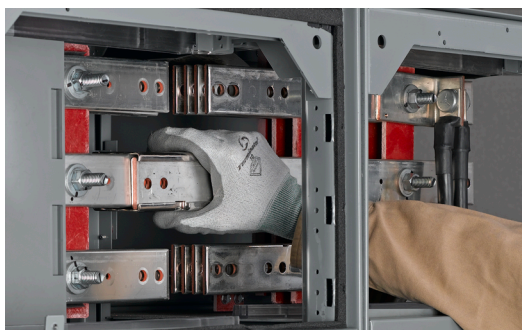
Figure 54 - Align the Splice and Bus Holes
