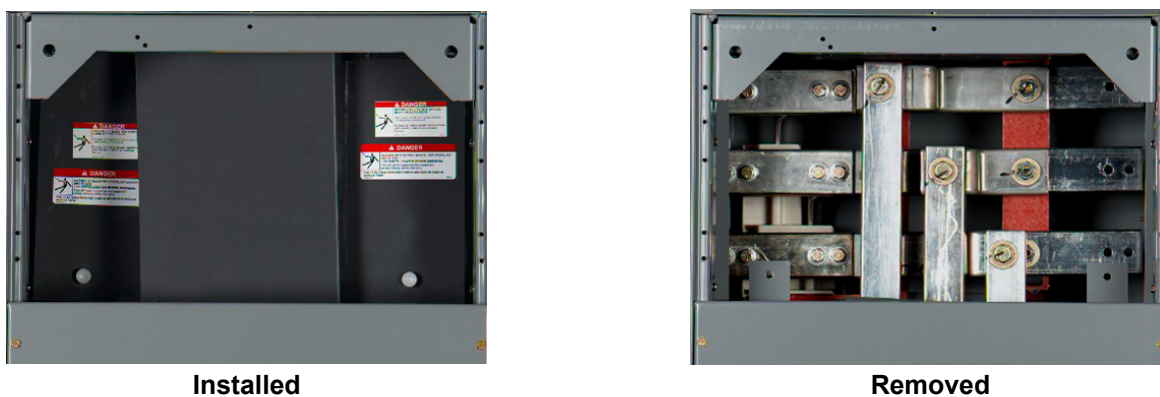
Figure 159 - Barrier Installed and Removed
