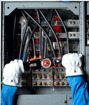
Figure 87 - Main Lug Compartment Torque Connection
