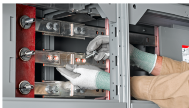
Figure 36 - Move and Align the Splice Bar to the Bus Holes
