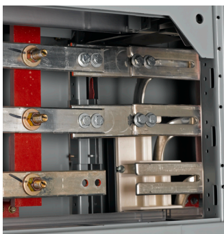
Figure 34 - Incorrect Application of Single-Bar Splice on Fork-Type Bus
