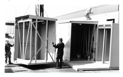
6. Using a crane, set the second aisle section onto the concrete pad approximately 12 inches (305 mm) from the section in place.
