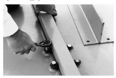
Figure 24 - Plugging Holes with Bolts and Seal Washers
