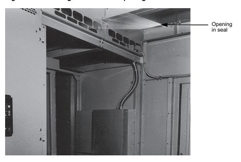
16. Remove the lifting lugs located on the roof of the switchgear and aisle (Removing Large Lifting Lugs, page 29 and Removing Small Lifting Lugs, page 29). Plug the holes with the 1/2-13 inch bolts and seal washers (Plugging Holes with Bolts and Seal Washers, page 30) furnished with each shipping section.
