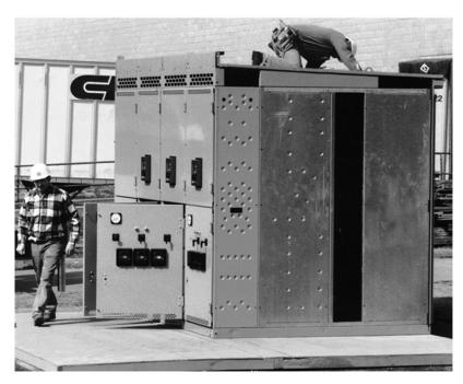
11. Install the equipment space sections (see Securing Equipment Space to Switchgear, page 22). Equipment space sections are designed similarly to switchgear units and can be unloaded and installed in the same manner.
