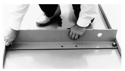
Figure 23 - Removing Small Lifting Lugs
