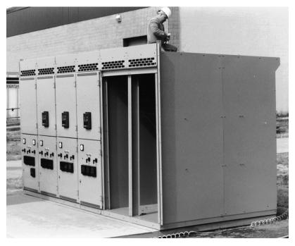
12. After the switchgear and equipment space sections have been installed, verify that all sections are aligned accurately, and that the bases and roof lines are level. Use a water level and a straight edge.
