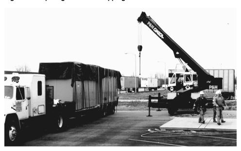
2. Unload the switchgear shipping sections from the delivery truck. The shipping sections are designed to be lifted by a crane. Attach a sling to the lifting lugs on the roof of each of the shipping sections as shown in . A spreader bar may be necessary to maintain proper lifting angles. If a crane is not available, contact Schneider Electric for special arrangements for unloading the switchgear sections.
