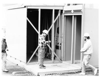
3. Attach the aisle section to the switchgear by bolting each bay's aisle roof support bracket to the front of the switchgear and by bolting the aisle roof to the switchgear roof, using the supplied 3/8-16 x 1.0 inch bolts (Anchoring Aisle Roof Support Bracket to Switchgear, page 24).
