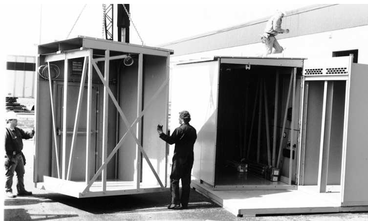
Figure 15 - Moving Sections with Braces in Place
