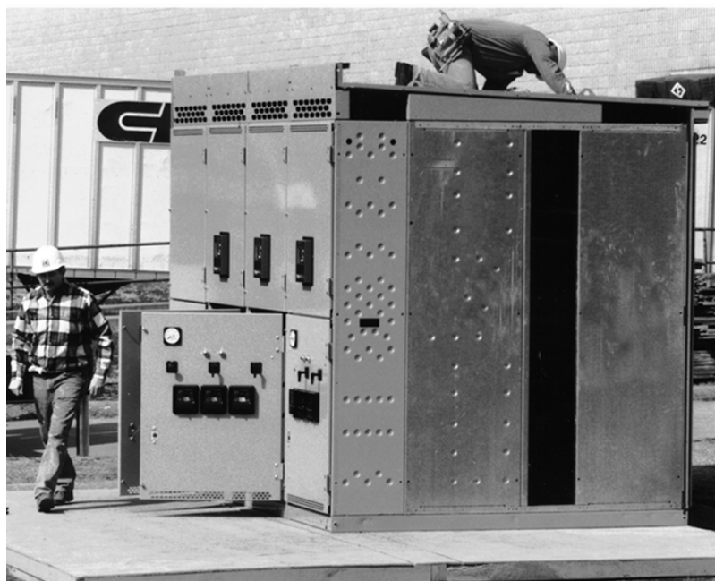
Figure 9 - Securing Switchgear Sections
