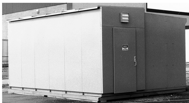
Figure 17 - Switchgear with all Sections in Place
