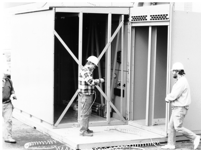
Figure 12 - Aligning Aisle with Switchgear Section
