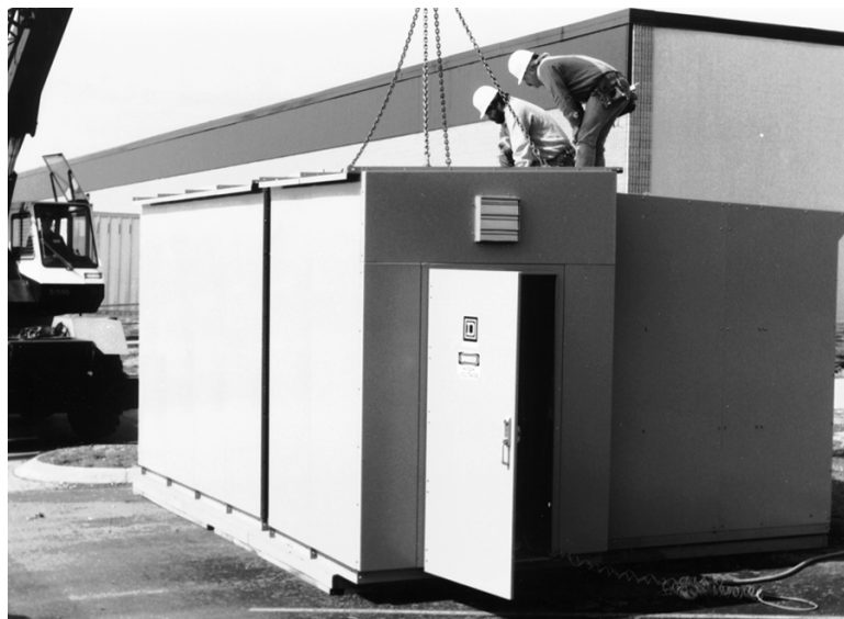
Figure 16 - Placing Second Aisle Section
