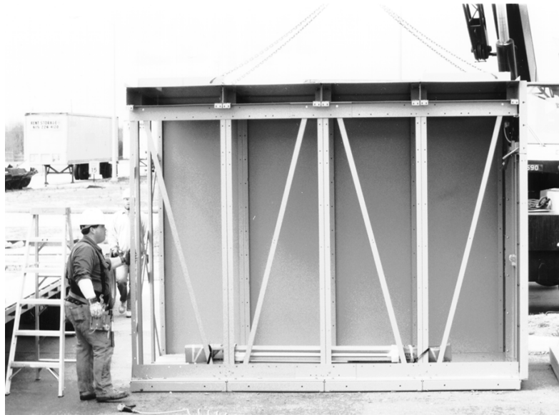
Figure 11 - Braced Front Aisle Section
