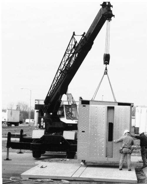
Figure 7 - Placing First Section
