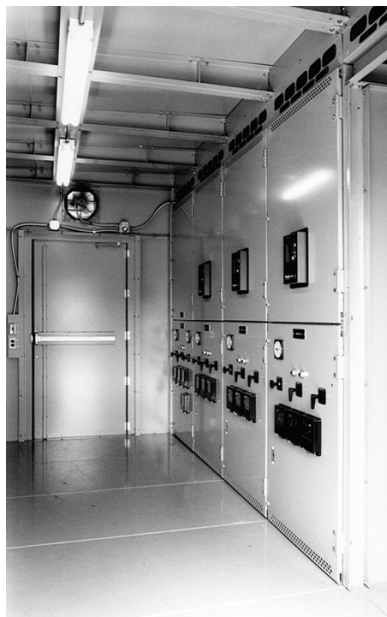
Figure 29 - Lights, Receptacle, and Fan
