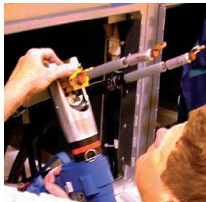
Figure 61 Mount cable lug
