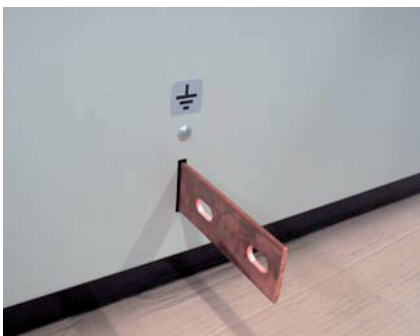
Figure 58 Connecting point of switchgear earth bus to building earth
