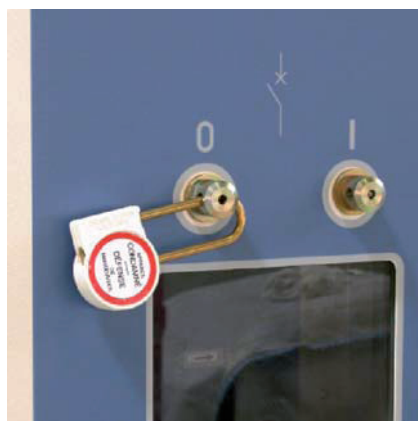
Figure 35 Manual switching OFF of circuit breaker locked by padlock
